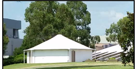
Photograph 6 – Detached toilet block
